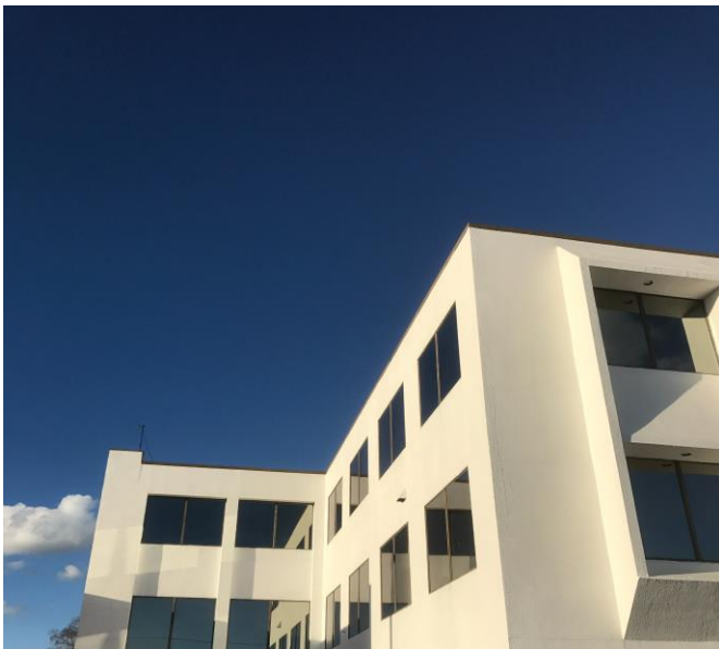
Sil-Wall-5001 (white) was used on the building above.
